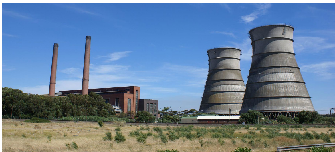
A decommissioned coal-fired power station in Cape Town, South Africa. © Danie van der Merwe via Flickr
